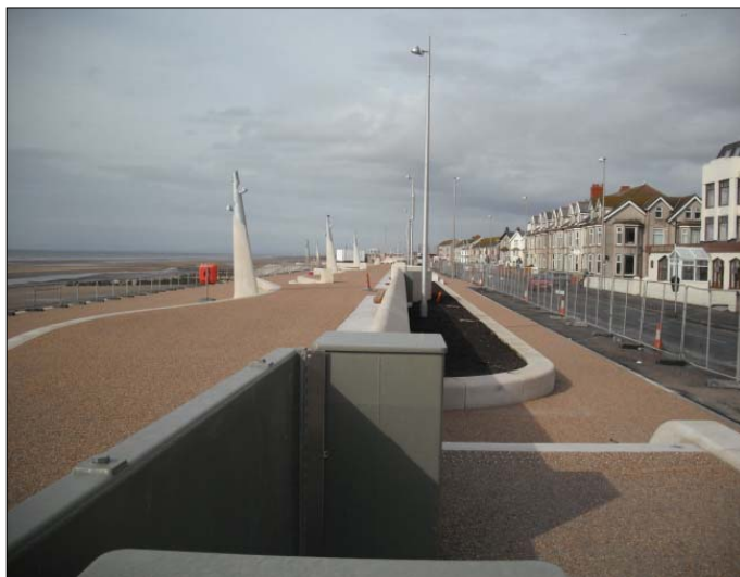
View looking north of the works looking along the sea wall.
