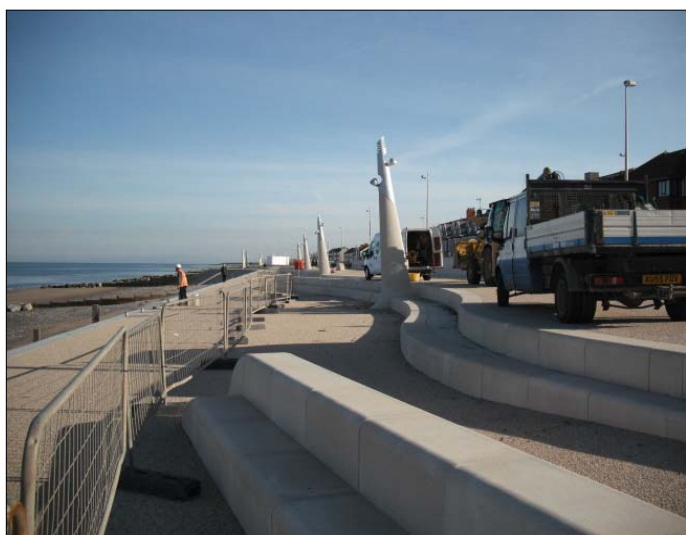
View looking north of the works along the lower promenade.
