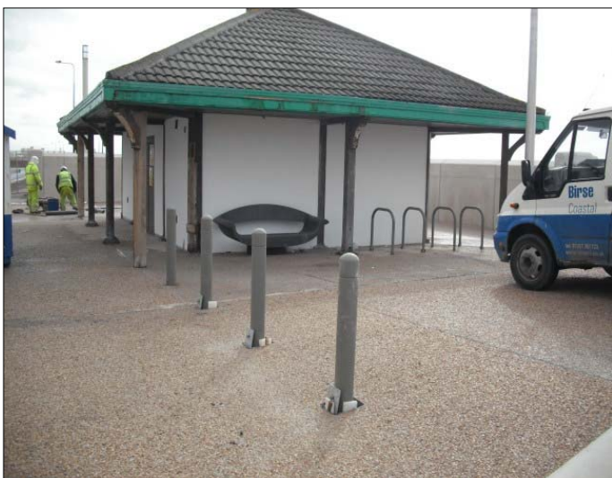
Bollards, benches and cycle racks installed around the pumping station.
