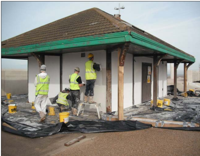
Rendering to the United Utilities pumping station walls being complete.
