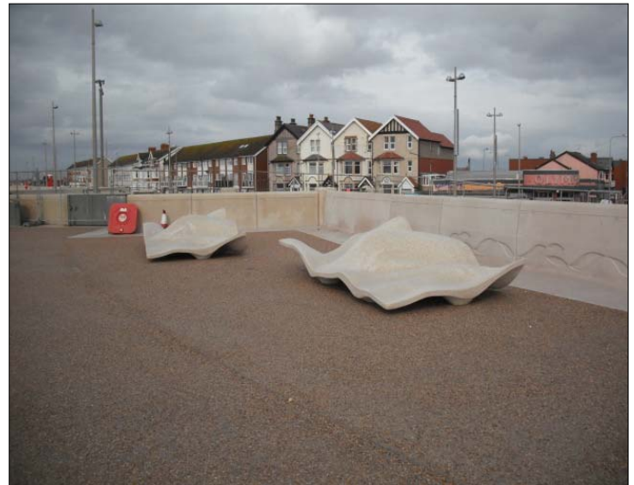
This phase of works seating includes the Escofet Lungomare seating above.
