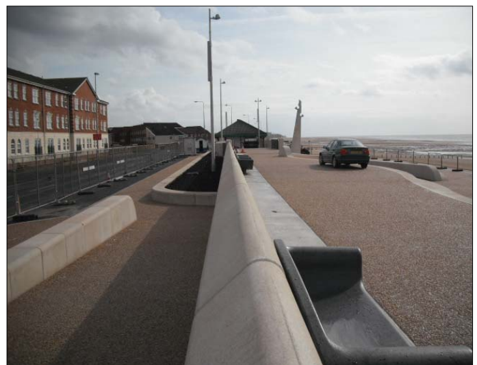
View along the sea wall showing both the sea side promenade and the highway side footpath and landscape strip.
