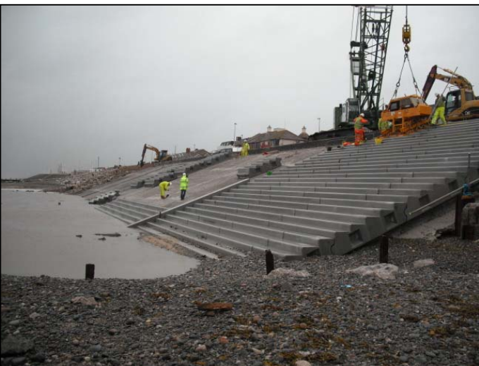
Last revetment unit in top row of panel 10 being placed.
