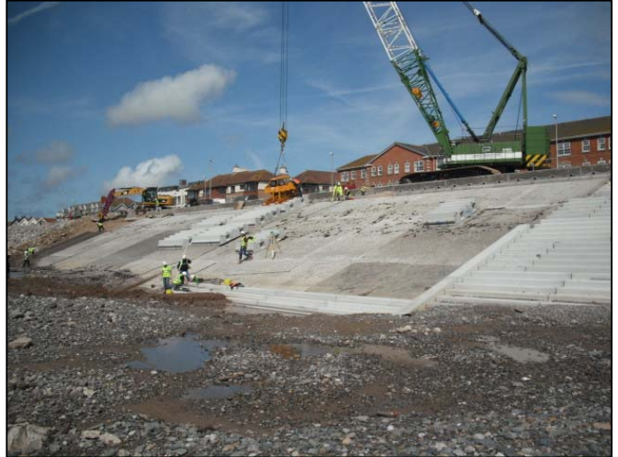
Lower row of units being completed in panel 9.
