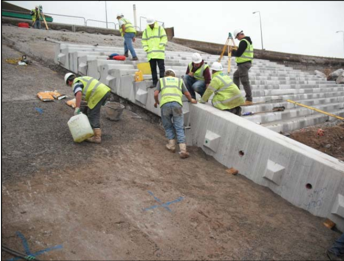
Lower spine beam between panel 9 & 10 being placed.
