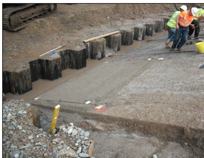
Screed and packers placed to line and level.
