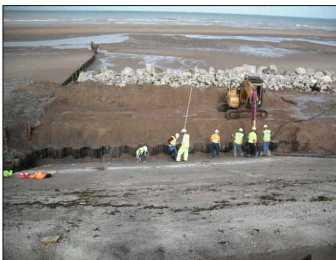
Setting out of the first revetment being carried out.
