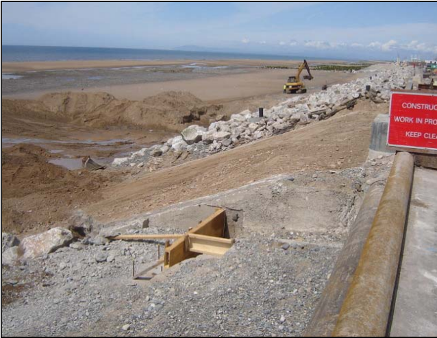
Southern most bay filled, compacted and trimmed to level ready to receive concrete.
