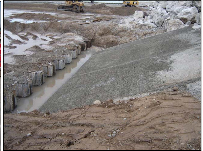
Bottom pour of southern most bay completed ready for placement of pre-cast concrete revetment units.
