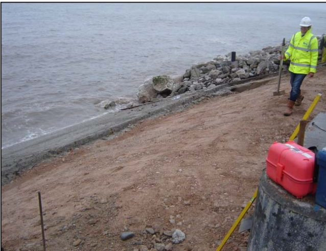
Middle pour of southern most bay completed with top section filled, compacted and trimmed to level.
