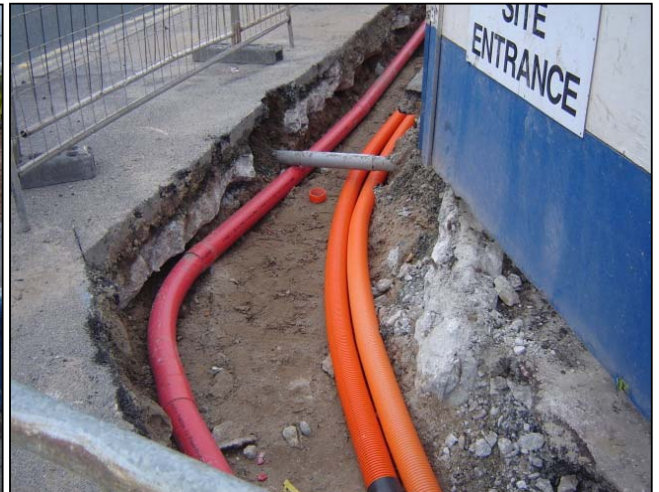
Electric and lighting cable ducting being installed around the pumping station.
