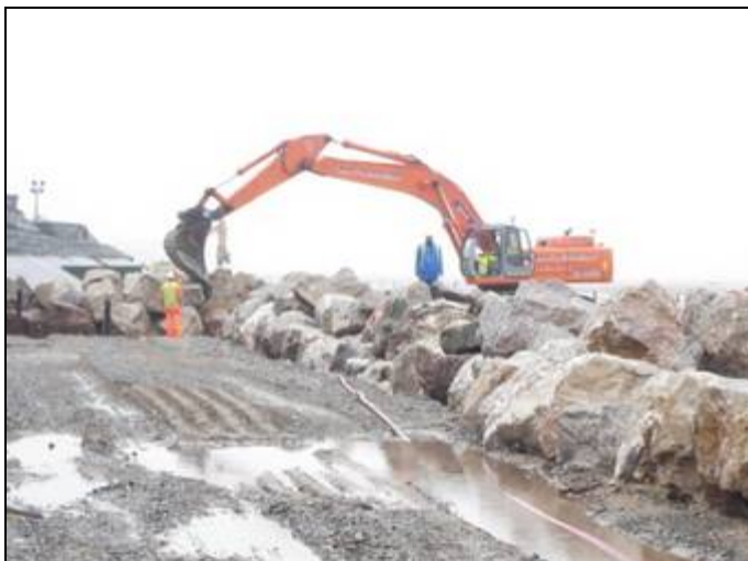
Rock armour being placed on the beach.
