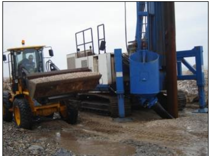
The rig hopper being loaded with stone.
