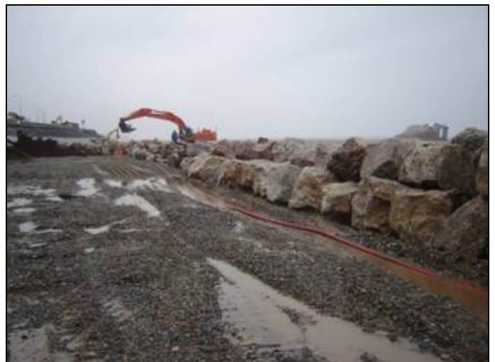
Rock armour in place.
