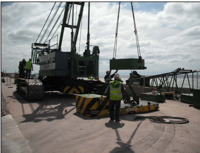
Crane being assembled.
