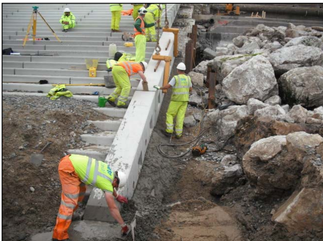
Southern most spine beam being installed.
