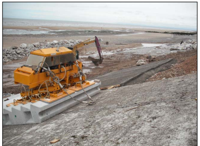
Middle third of revetment preparation completed to panel 7.
