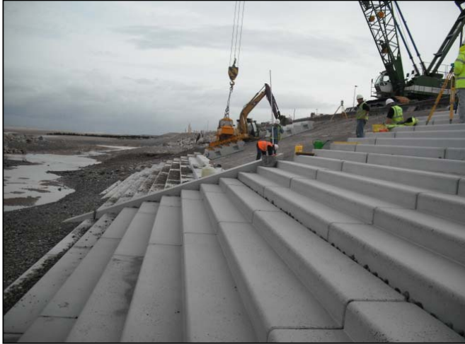
Continuing precast revetment installation to bay 9.
