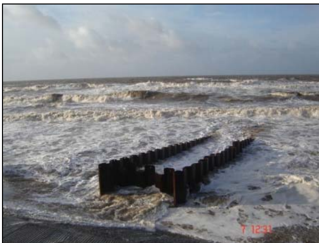
Slade extension under construction
