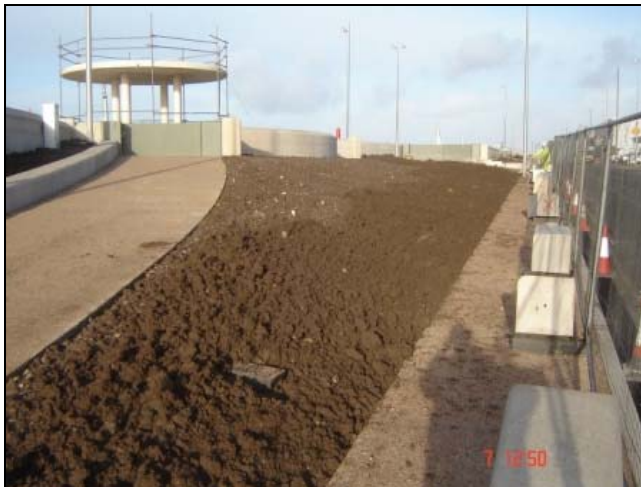
Landscaping works alongside North Promenade
