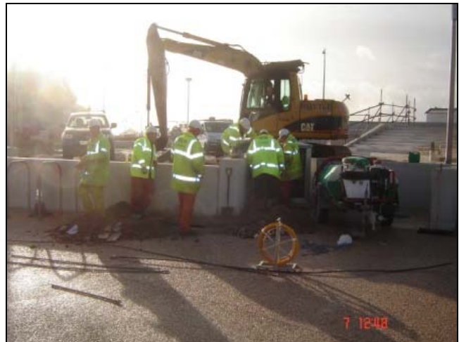
Installing electrical cabling to recreational area
