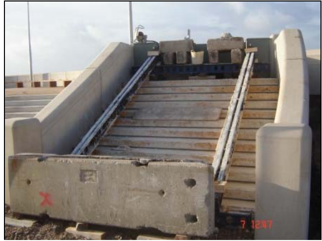
The promenade access steps to the north of the plaza area
