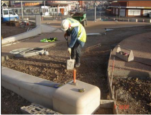
Preparation works to the pedestrian areas at the plaza area
