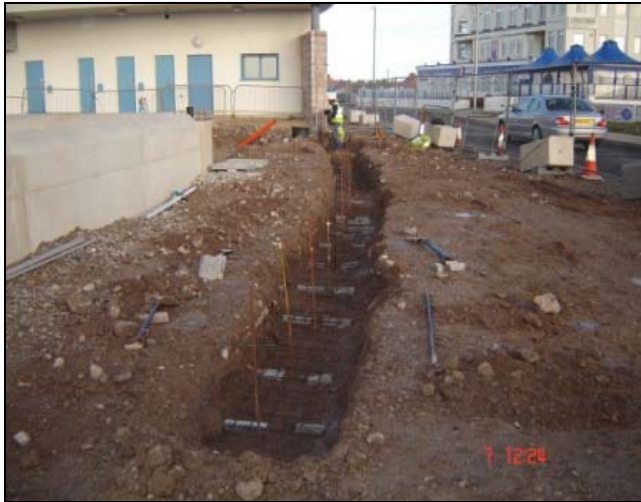
Forming the foundations for the new roadside wall
