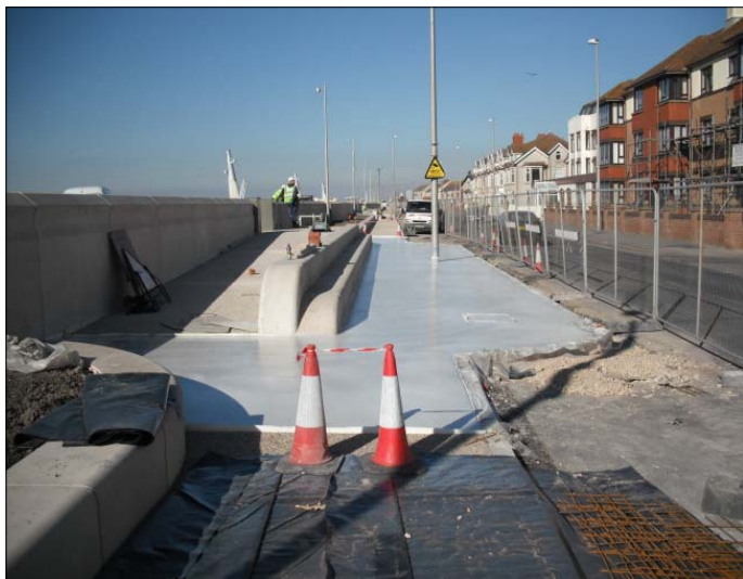
Footpath pavement slab concrete just poured with retarder applied to surface.
