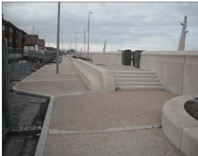
Completed footpath around storm gate pedestrian access point.
