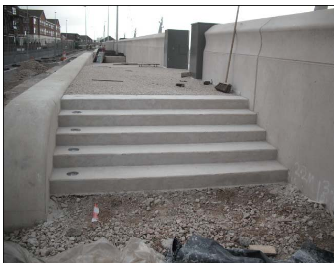
Storm gate pedestrian access steps.
