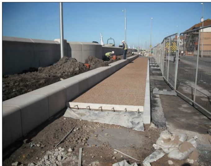
Completed section of public footpath.
