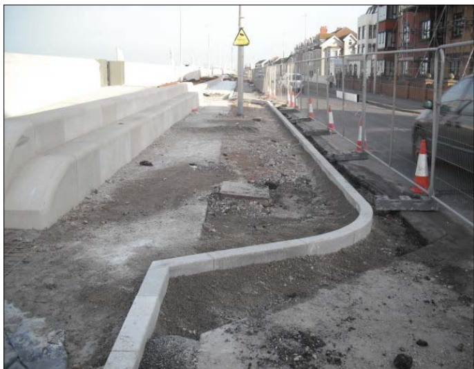
Kerbing installed adjacent to a pedestrian access point.
