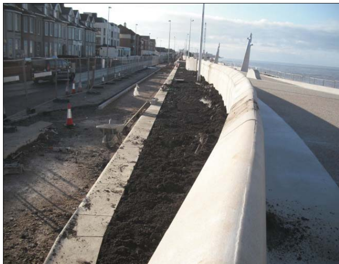
Topsoil to the raised landscape strip.
