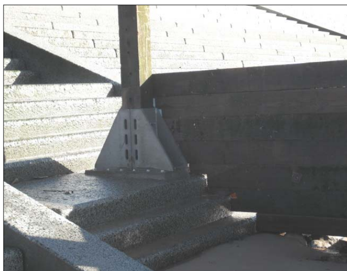
Groyne post repair adaptor.
