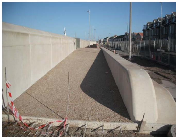
Storm gate pedestrian access ramp completed pavement.
