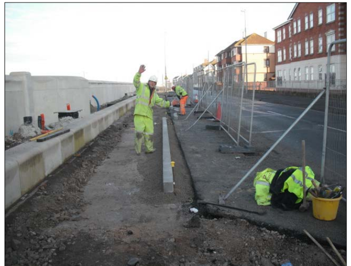
Installation of kerbing adjacent to highway commencing.
