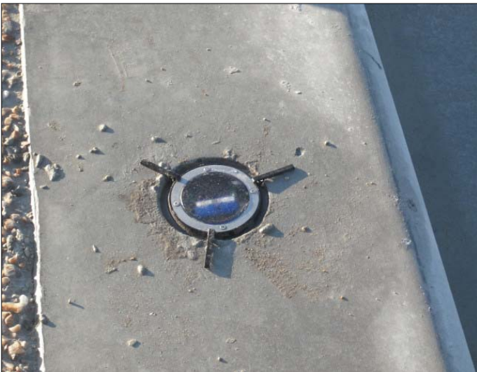
Solar powered ground edge lighting installation.
