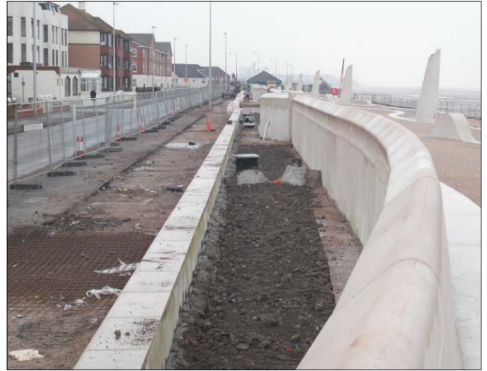
Coarse sub base placed to base of landscape strip.
