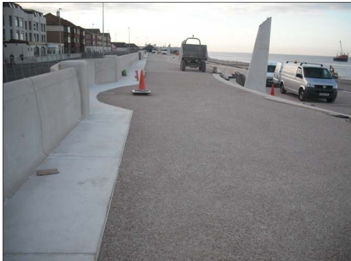
Upper promenade exposed aggregate pavement slab.
