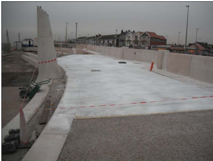
Pavement slab with retarder applied to surface.
