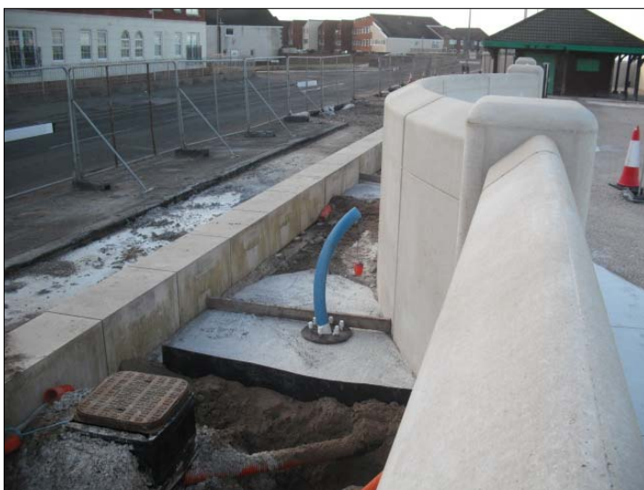
Shelter pad foundation.
