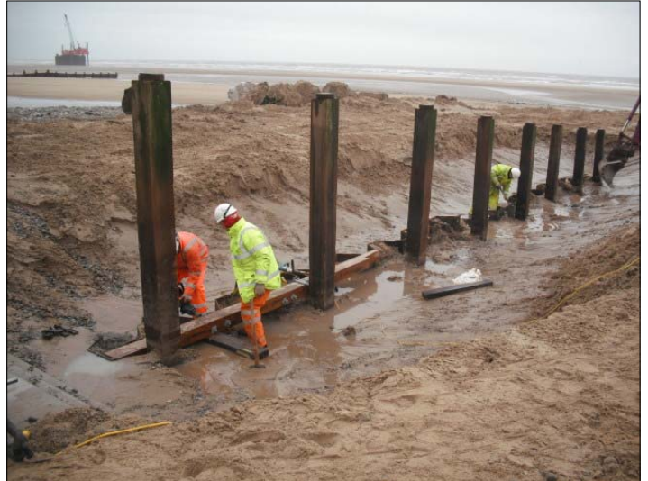
Timber waling connecting groyne post to steel sheet piles.
