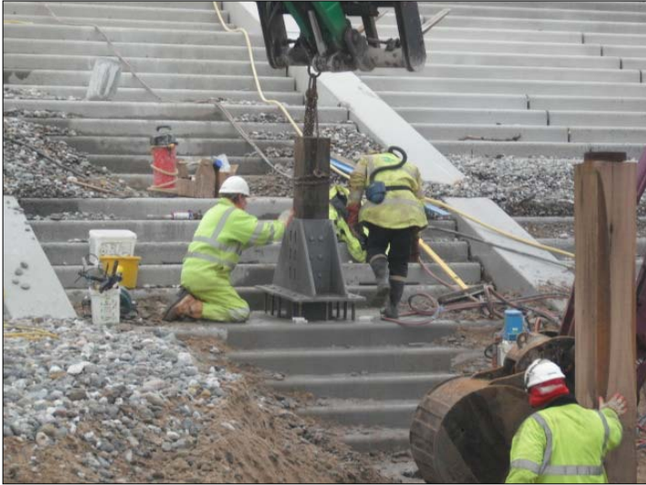
Revetment groyne post being installed.
