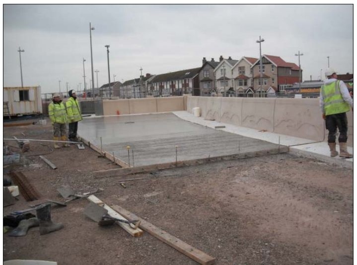
Promenade pavement slab being poured.
