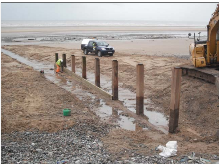
Groyne boarding being bolted to posts..
