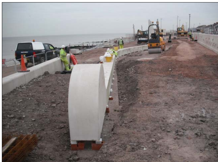
Last units of split level promenade precast wall units placed.
