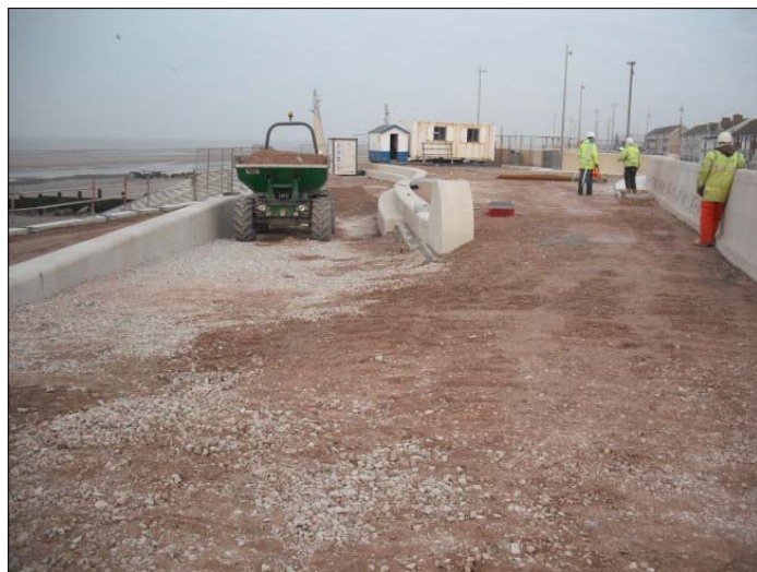
Fill and compaction to promenade formation level complete.
