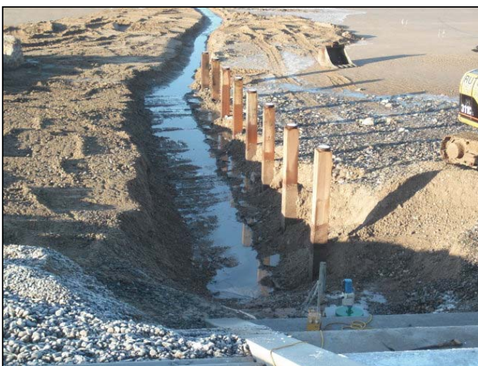
Excavation adjacent to groyne to allow timber works.
