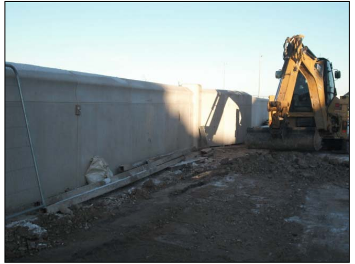
Highway side of completed precast rear wall placement.
