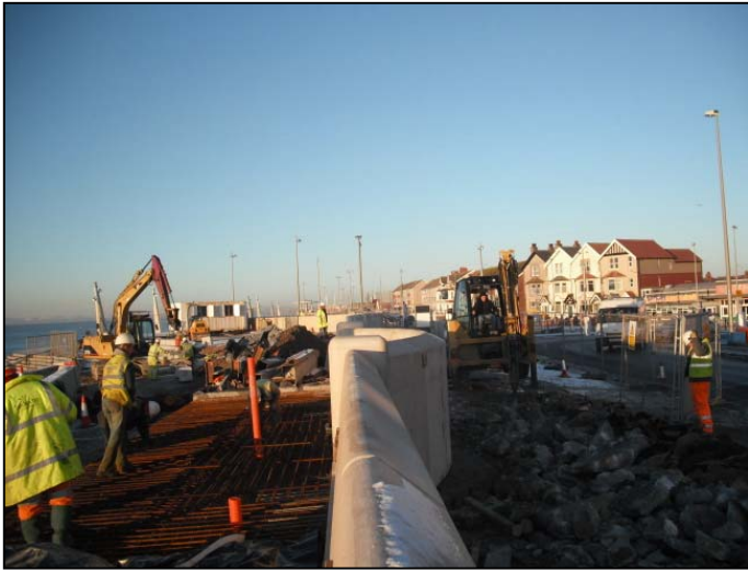
Remaining precast rear units placed and reinforcement to base being fabricated.
