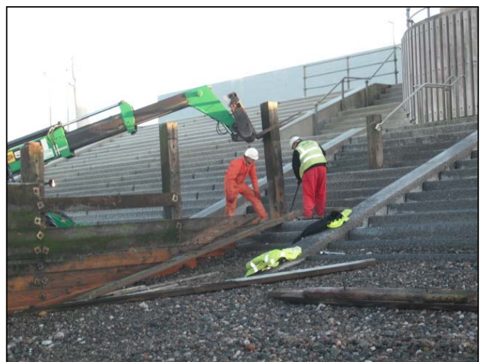
Remedial works to phase 2 groynes.
