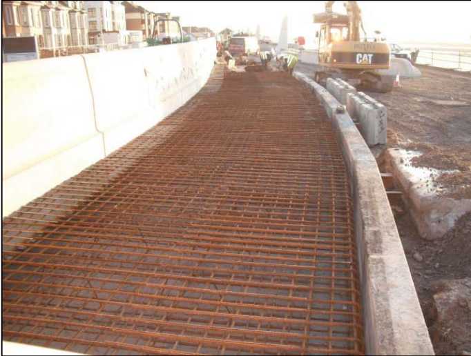
Reinforcement in place to the rear wall base ready for concrete.
