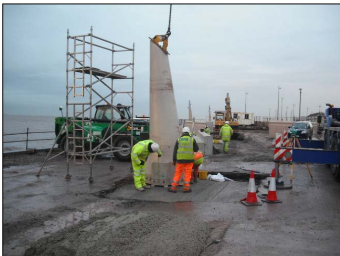
Final feature lighting column being set in position.
