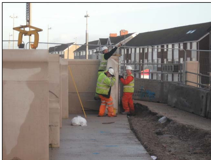
Final section of precast wall units being installed.
