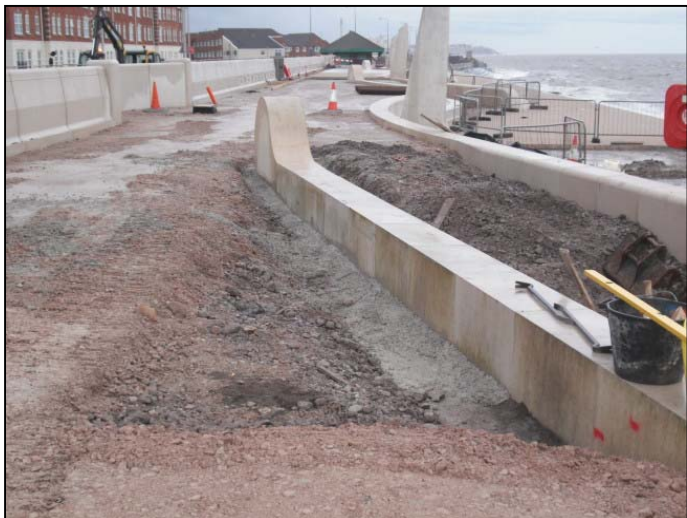
Last upper units of wave 3 installed.
