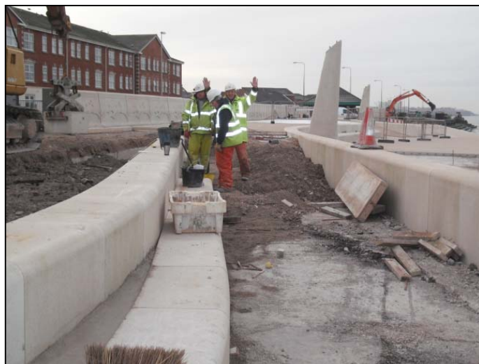
Last remaining units of wave 4 being installed.
