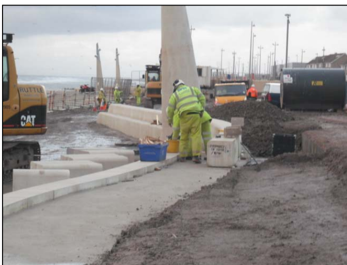
Upper intermediate units of wave 3 being installed.
