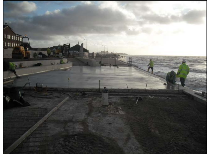
Lower promenade pavement being finished.
