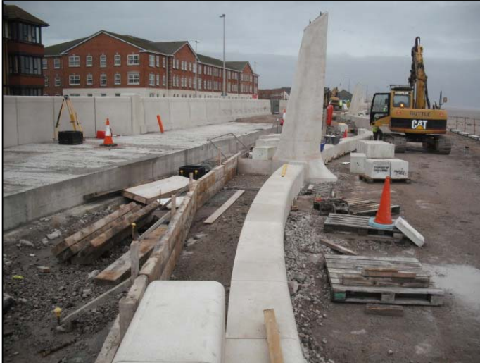
Intermediate wave 4 walls being constructed.
