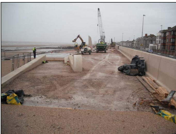
Upper promenade fill and sub base compacted ready for pavement pour.
