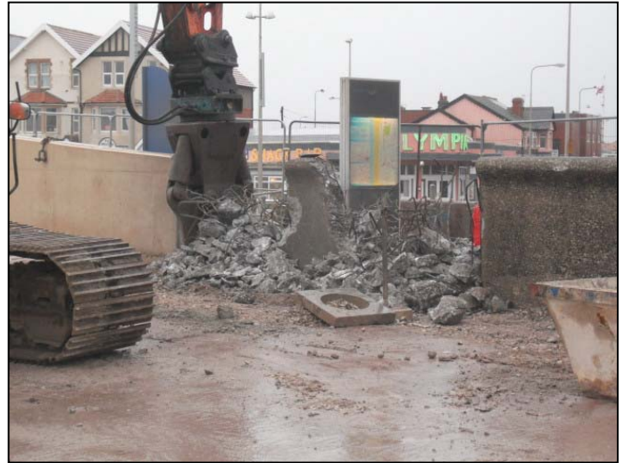
Last length of existing sea wall being demolished.
