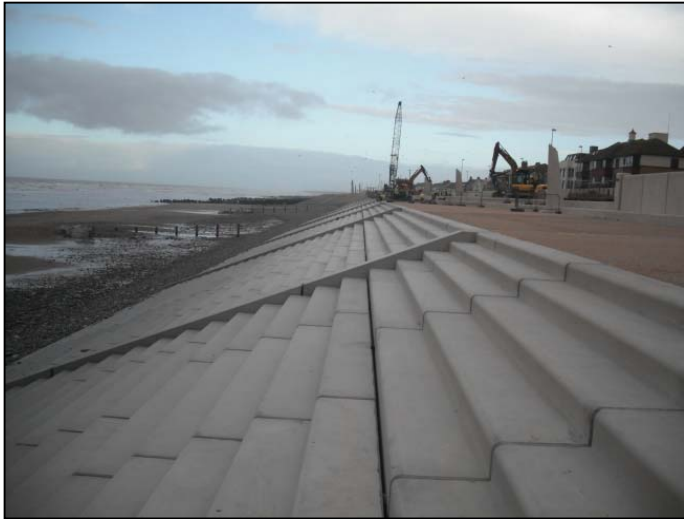
The completed revetment.
