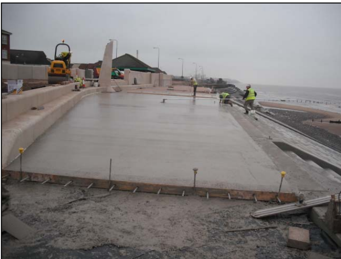
Lower level of exposed aggregate promenade concrete being finished.
