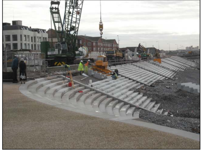
Last row of revetment units being placed.
