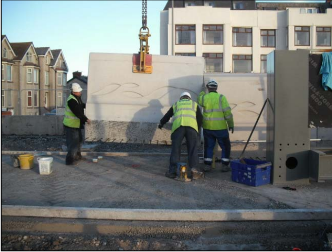
Precast rear wall unit being lowered into position.
