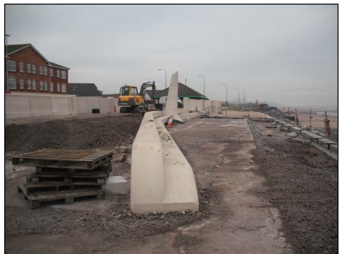
Wave 6 upper and lower intermediate walls complete.
