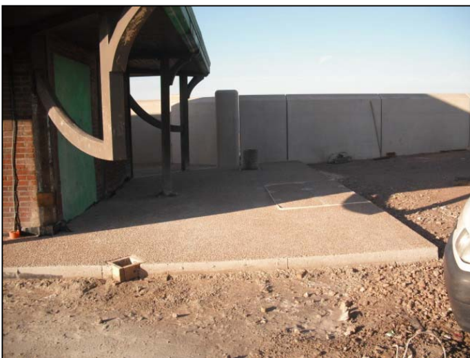
Part of pavement slab around pumping station complete.
