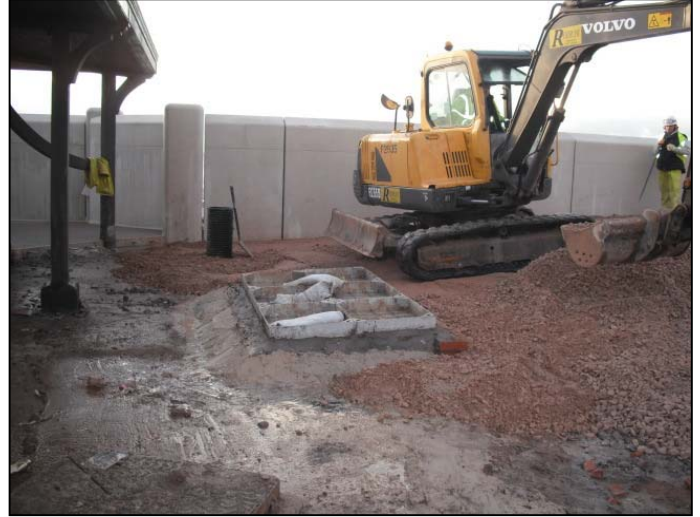
Southern storm gate access ramp formation being prepared.
