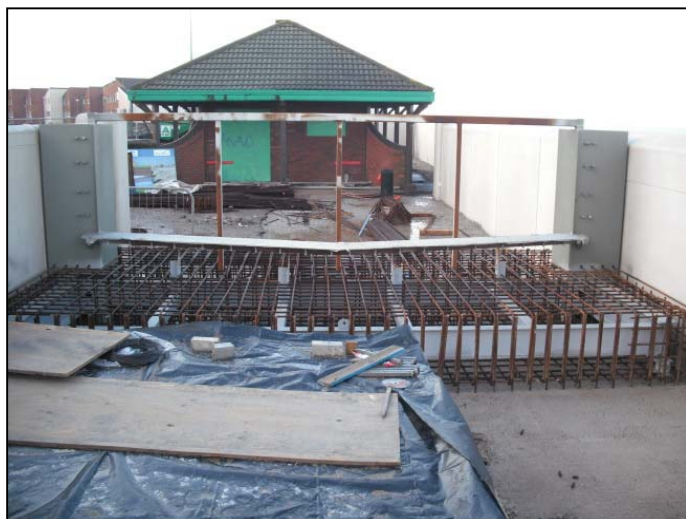
Storm gate reinforcement in place ready for in-site concrete base.
