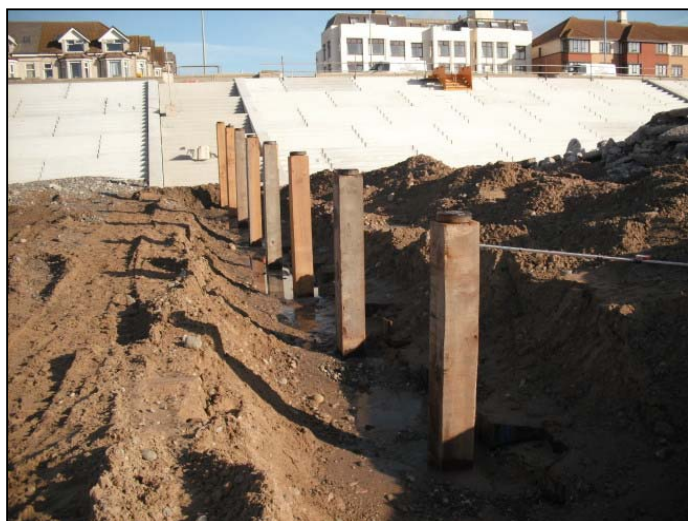
Groyne timber posts driven to level.
