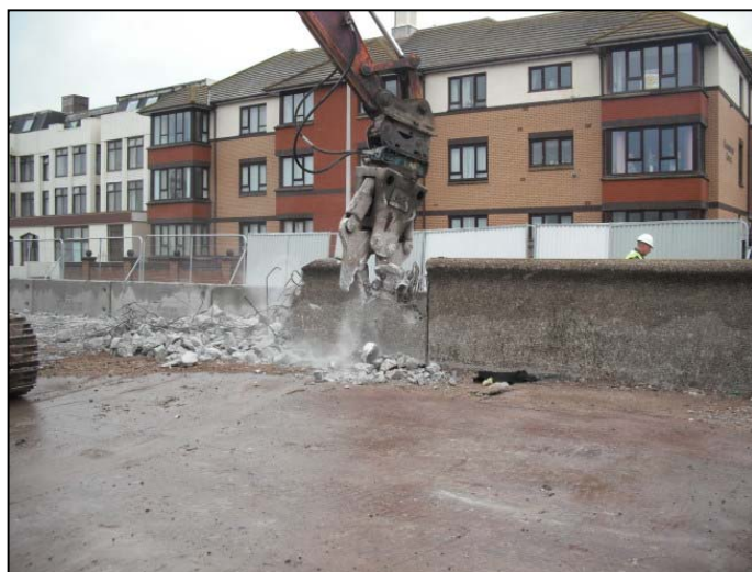
Existing sea wall being demolished with 'muncher'.
