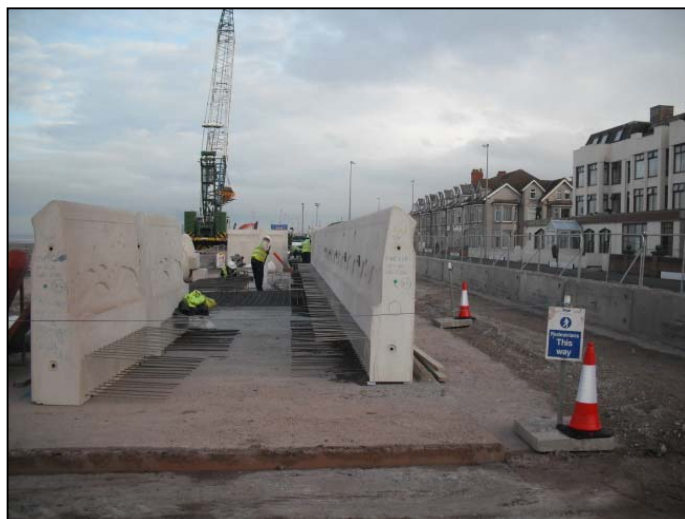
Continuing installation of pre-cast rear wall units.
