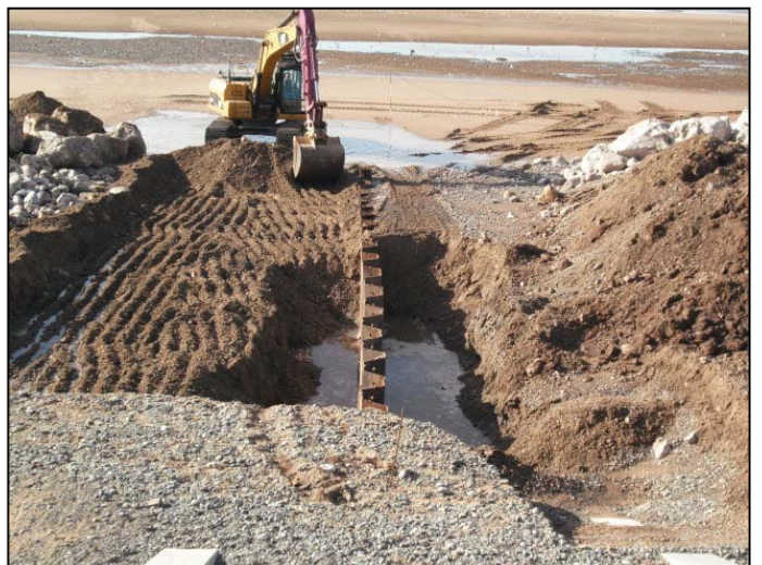
Groyne piling installed.
