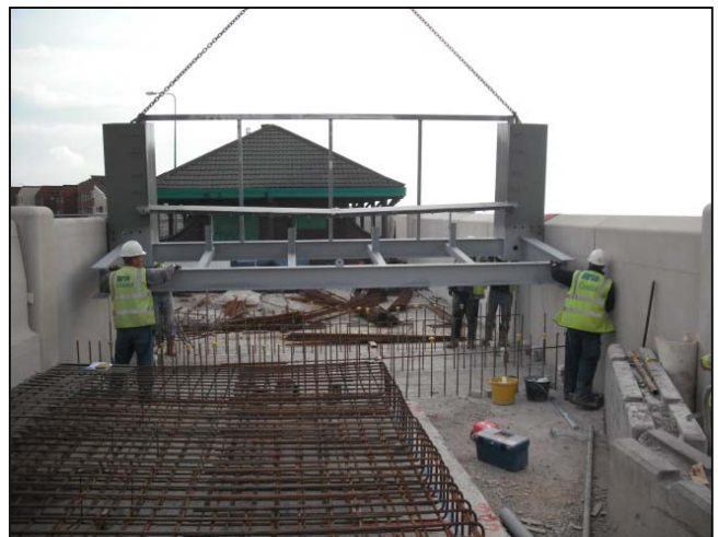
Storm gate frame being installed adjacent to pumping station.
