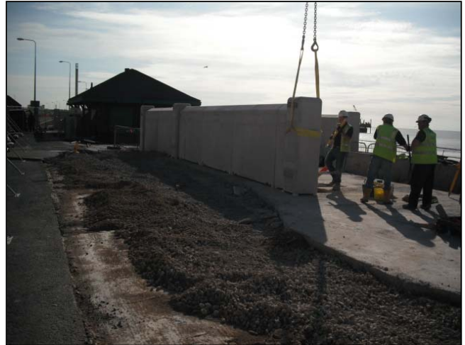
Pre-cast rear wall units being placed to line and level.
