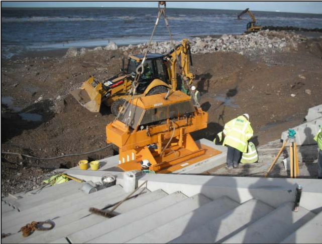
Lower pre-cast pedestrian access stepped unit being placed.
