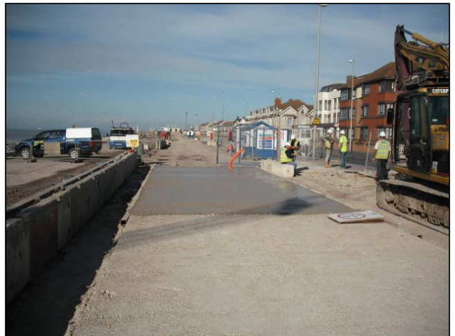
Blinding concrete to underside of rear wall and base slab.
