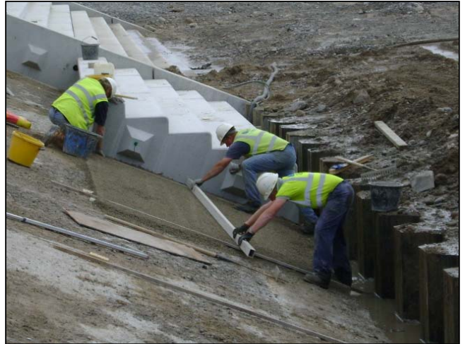
Revetment unit screed bed being levelled off.
