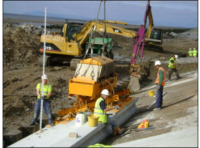
Revetment unit being checked for level.
