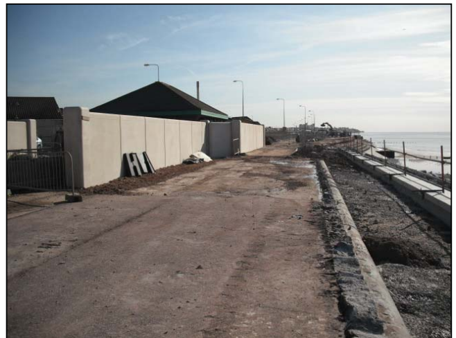
Wall units to rear of pumping station in position.
