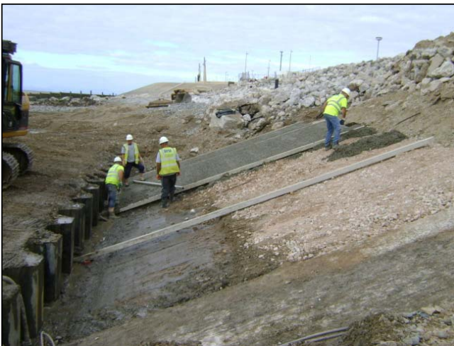
Lower section revetment foundation being prepared.
