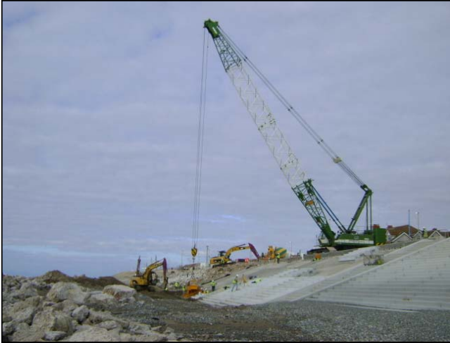
View from beach of revetment units being placed.
