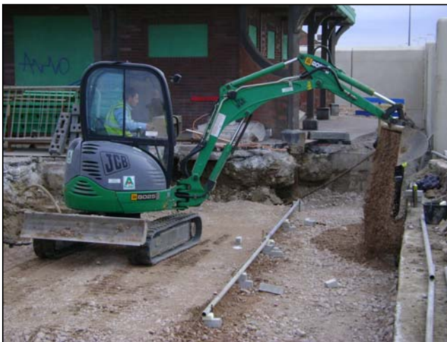
The ground is prepared to accommodate more wall units.
