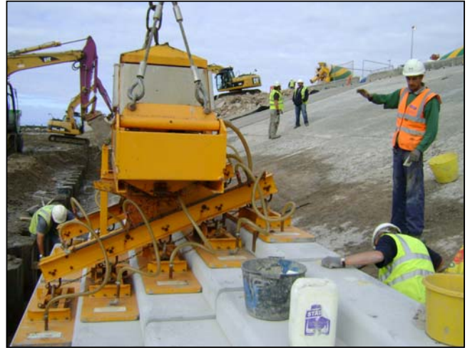
Pre-cast stepped revetment unit being lowered into position.
