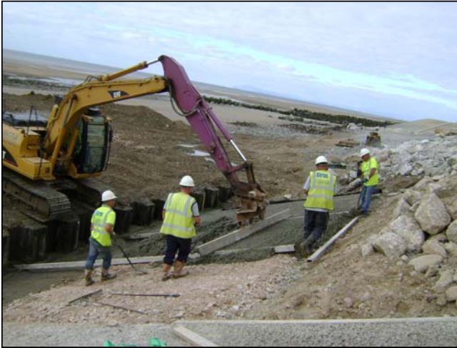
Concrete is placed to revetment slope.
