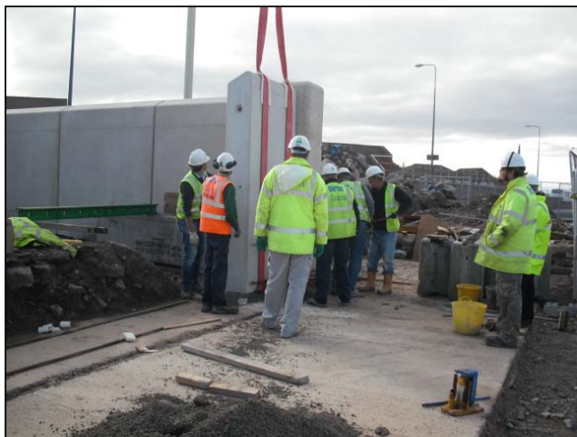
Precast wall unit being placed to correct line and level.
