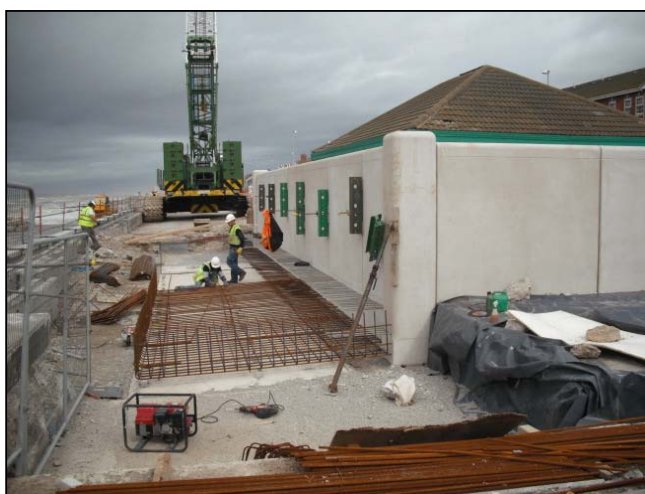
Reinforcement cage being fabricated to base of wall units.
