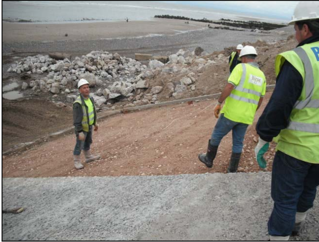
Last pour of panel 5 blinding being prepared.
