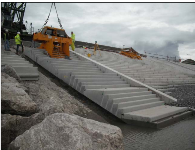
Steps showing vacuum lifter specifically for step units.
