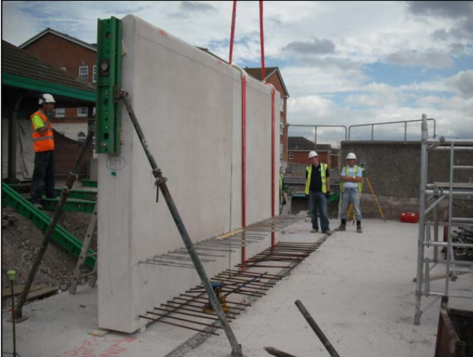
Precast wall units being placed along the southern boundary.
