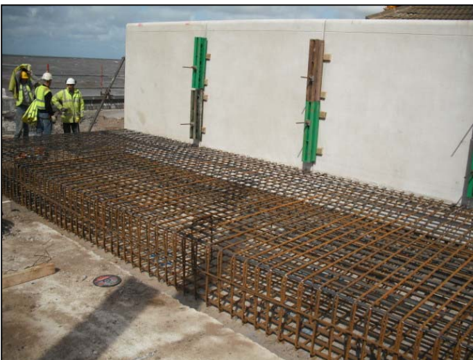
Slab reinforcement to rear wall
