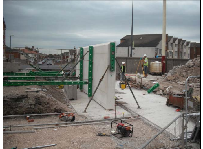
Precast wall units in place with temporary support system.
