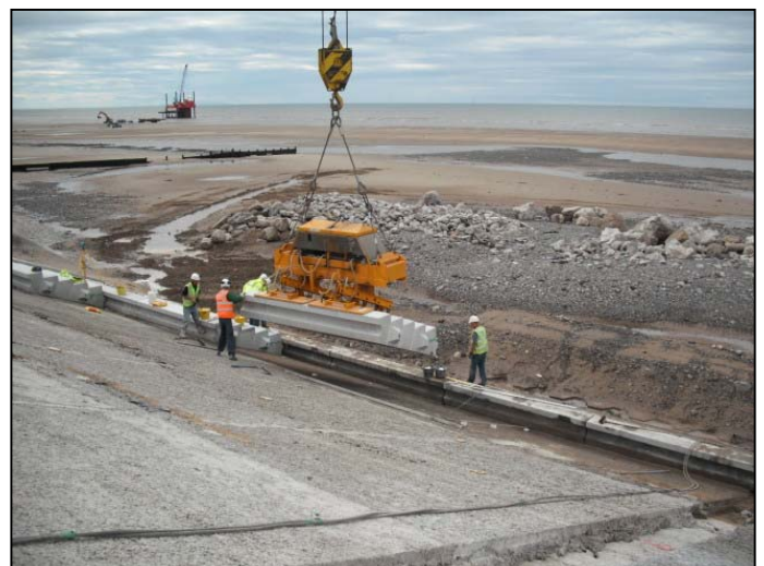
Installation of panel 7 revetment
