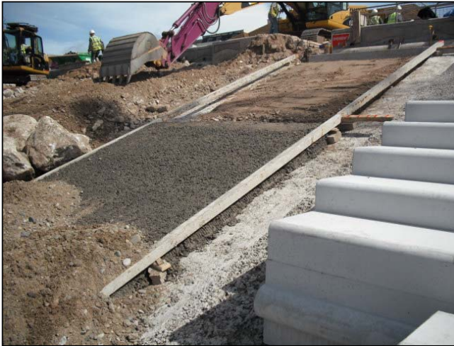
Blinding to upper section of access steps being placed.
