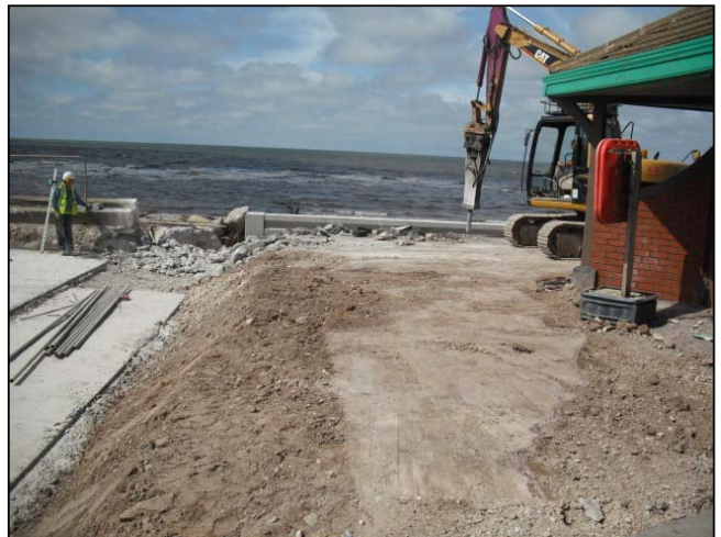
Parapet wall removed.
