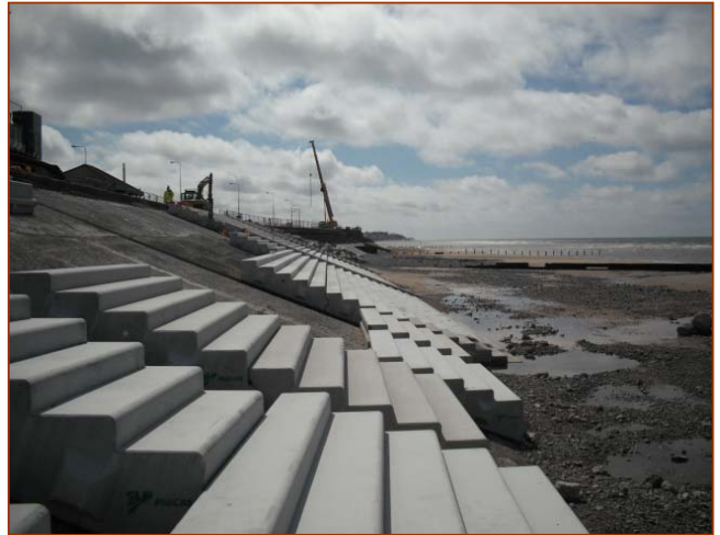
View looking south of revetment units placed to date.
