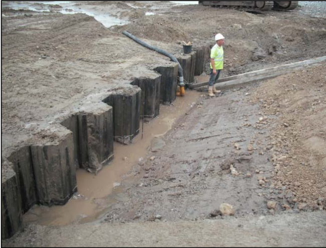
Lower pour being trimmed, filled and compacted to level.
