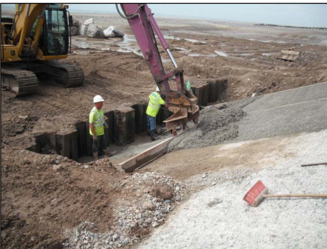
Machine adapted screed rail levelling concrete to profile.
