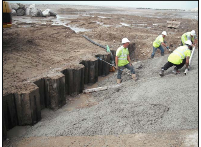
Blinding concrete being placed to lower pour.
