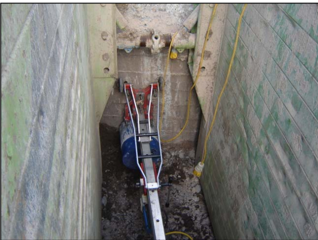
Diamond core drilling of existing seawall for drainage outfall.
