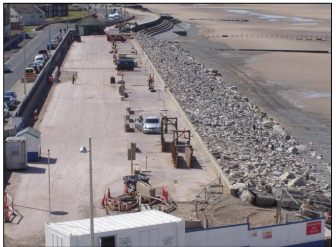
Aerial view of Phase 4b site.
