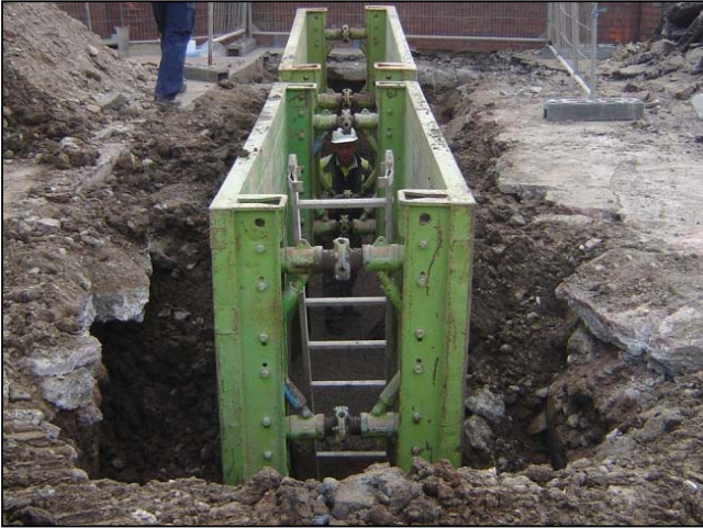
Trench box installed.
