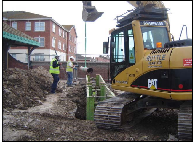
Length of drain being lowered into trench.
