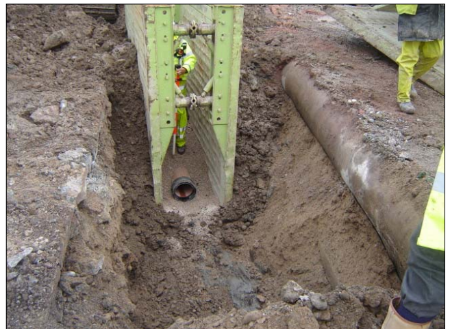
New drainage being installed.
