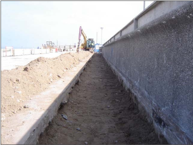
Last length of trench ready for ducting.
