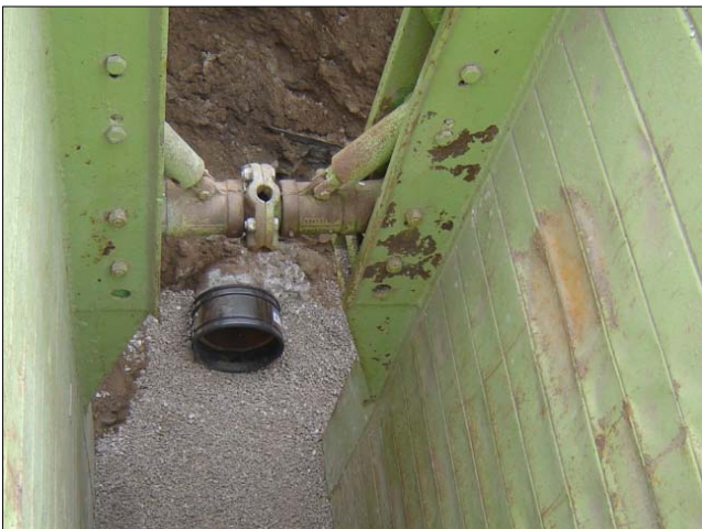
Existing drainage ready to receive new drainage within trench box.
