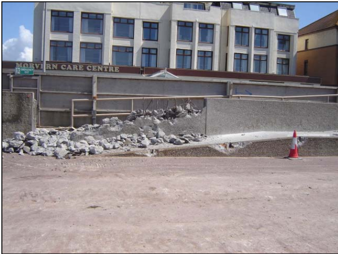
Pedestrian access ramp demolition.
