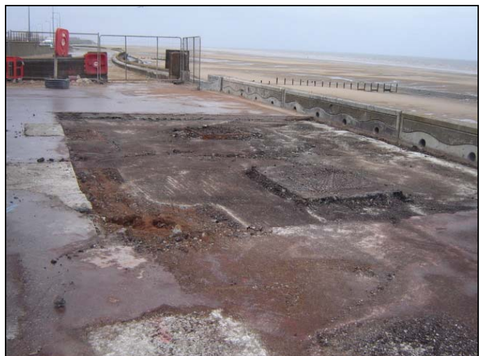
Surfacing of abandoned outfall chamber removed revealing chamber concrete roof.
