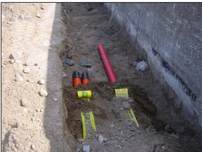
Lighting and electric cable ducting installation.
