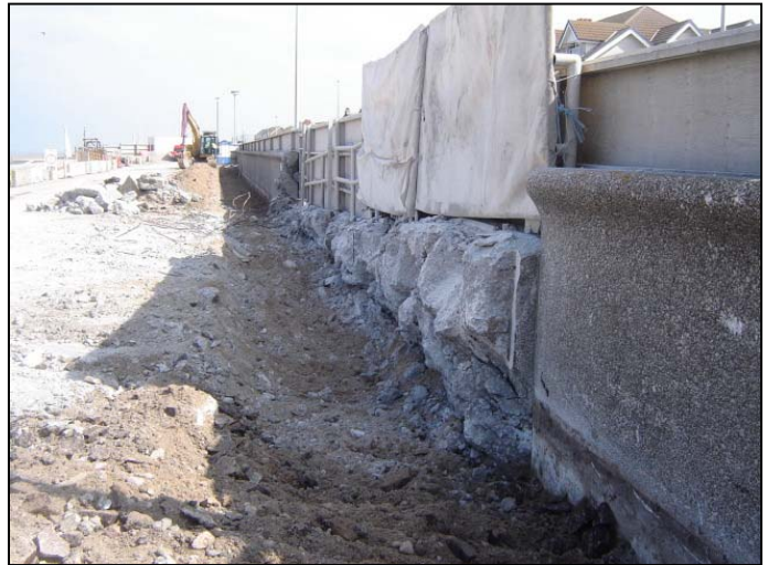
Completed pedestrian access ramp demolition.
