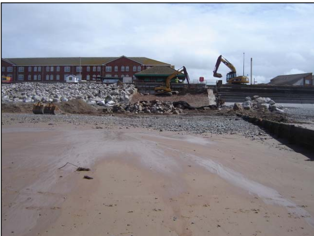
Southern end of works being completed.
