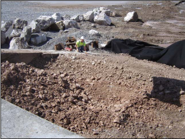
Southern-most bay being filled and compacted to level.
