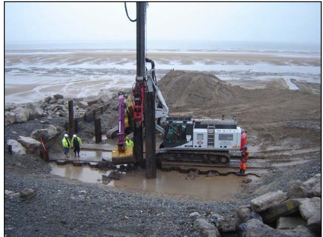
Southern 10metres of piles being re-driven.
