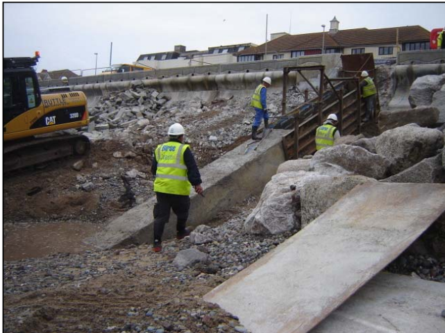
Final section of diaphragm wall concrete being prepared.
