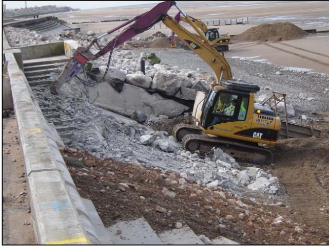
Last set of existing steps being demolished.
