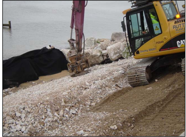
Fill material being compacted prior to loading material being placed.
