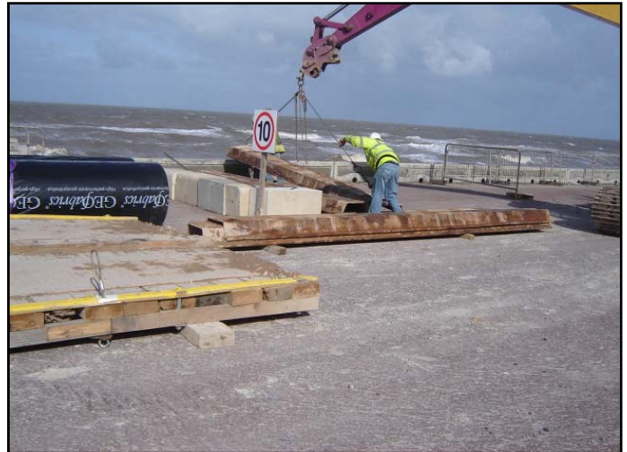
Installation of temporary bridge over the United Utilities storm tank.
