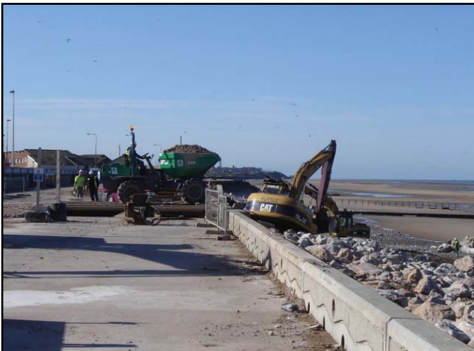
Temporary bridge being utilised for placing of fill material.
