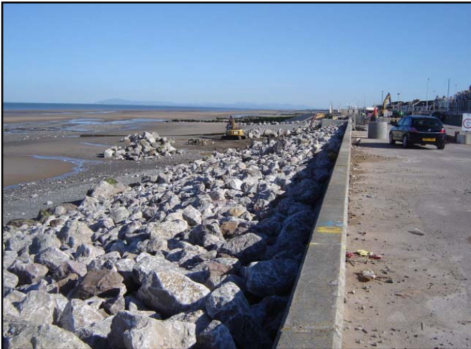
Completed filled bays topped with loading material.
