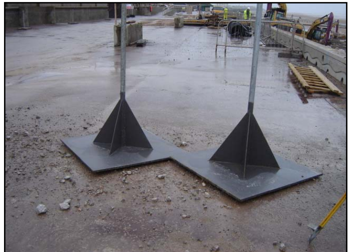
Settlement monitoring station prior to placing within the fill material.
