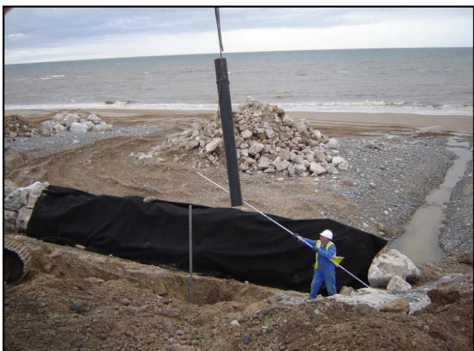
Installation of a monitoring station.
