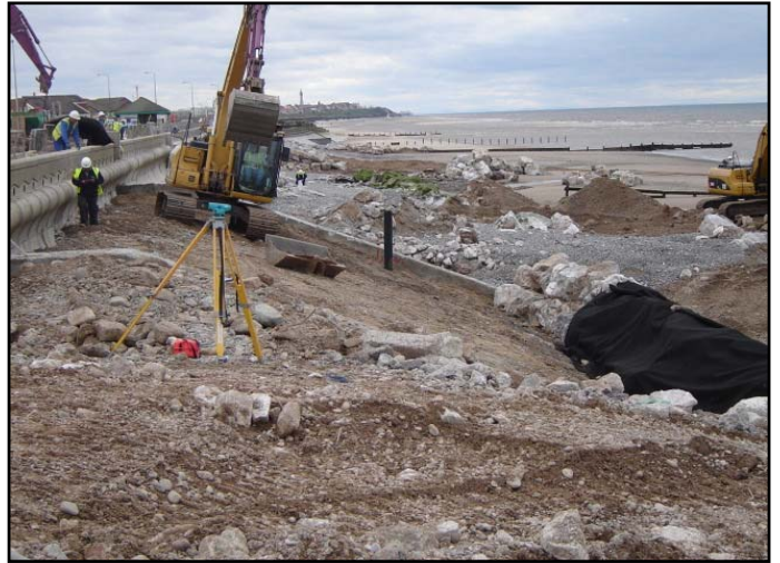
Northern bays being filled with imported fill material.
