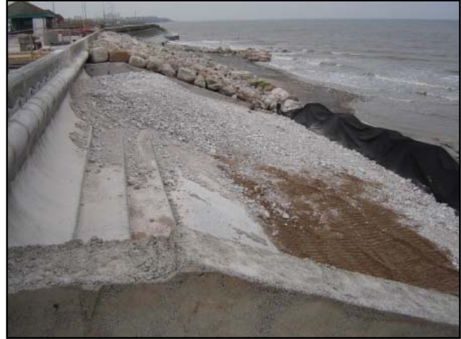
Completed and part completed bays.
