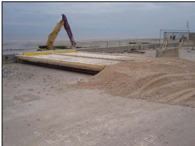
Temporary bridge over the storm tank buried beneath the promenade.
