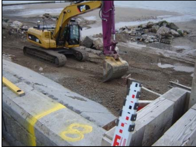
Preparation of bay prior to fill material being placed.
