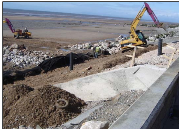
Beach material being placed on the fill material.
