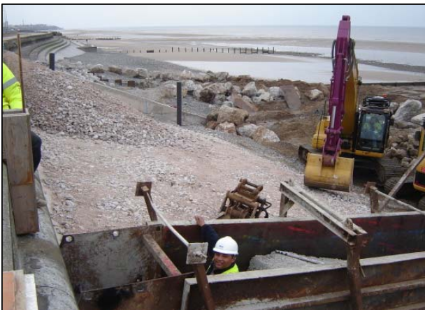
Graded fill being placed between diaphragm walls.
