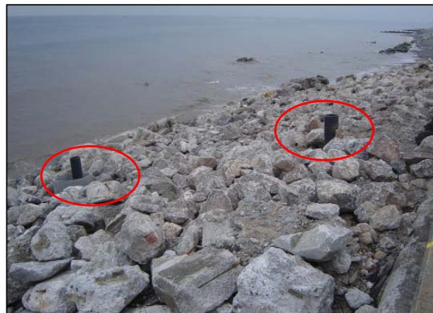
Settlement monitoring stations.
