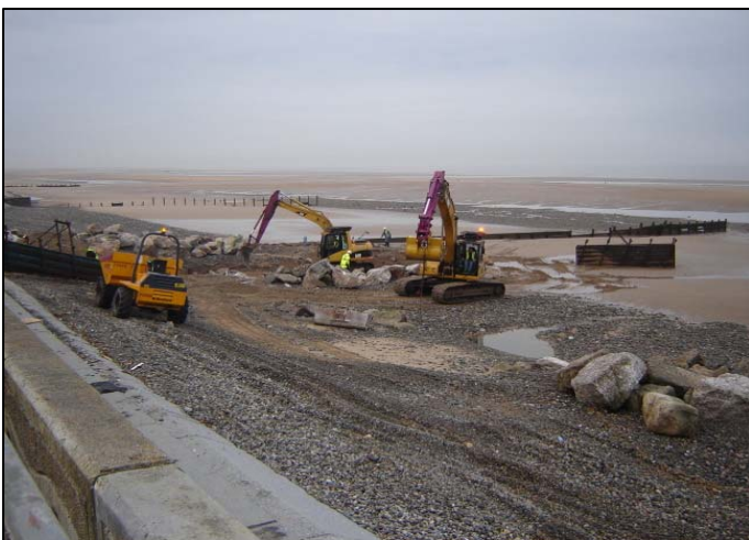
View of the diaphragm wall work location looking south
