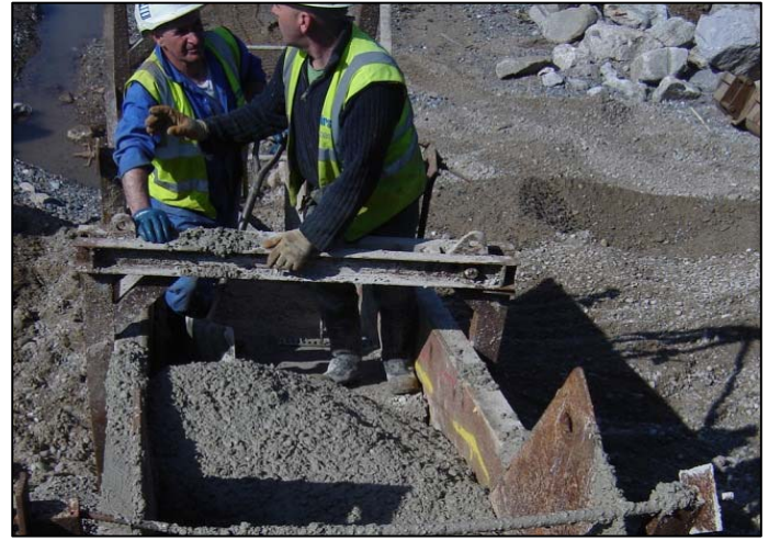
Concrete being placed in the upper section of diaphragm wall.
