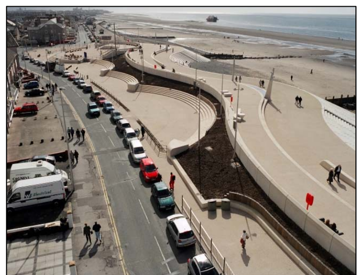
Completed phase 3 works
