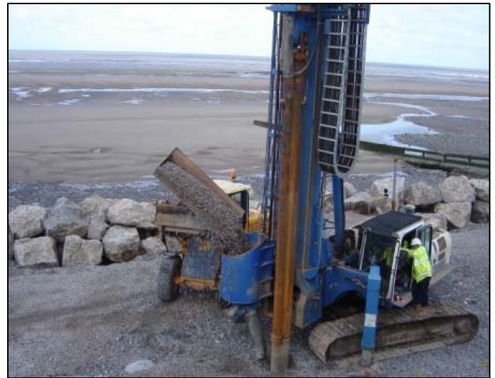
Placing of vibro stone column piles
