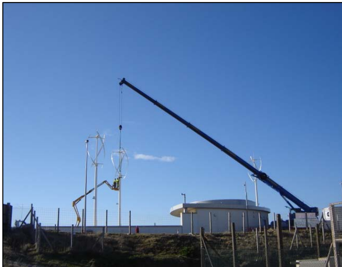
View of extent of crane reach
