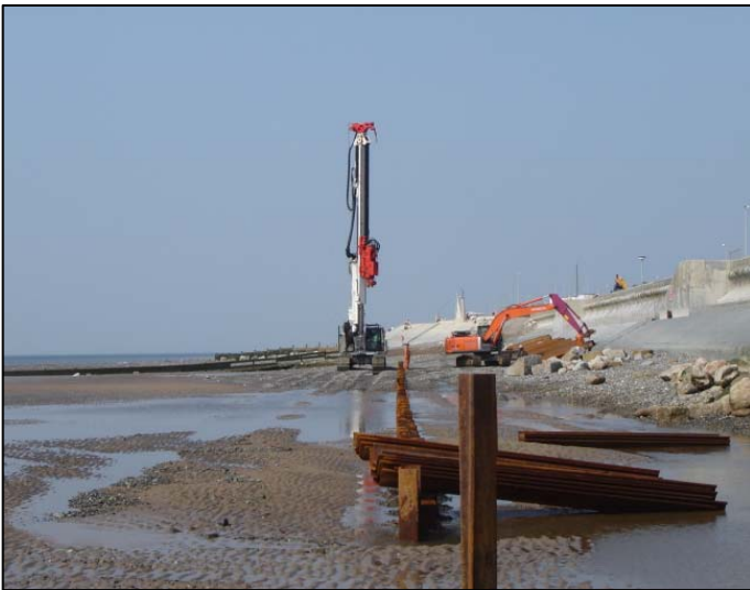
Steel piles along revetment toe line
