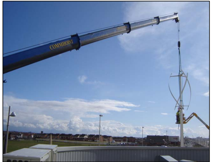
Turbine being mounted on to mast
