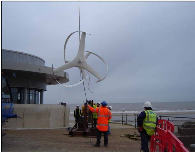
Turbine being lifted from its transportation frame
