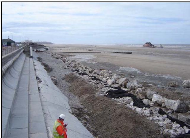
Rip rap protection of the stone piles.
