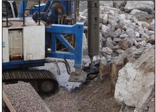
Close up of the piling rig water jet.
