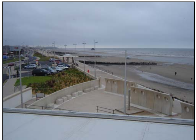
View from the cafe roof looking south.
