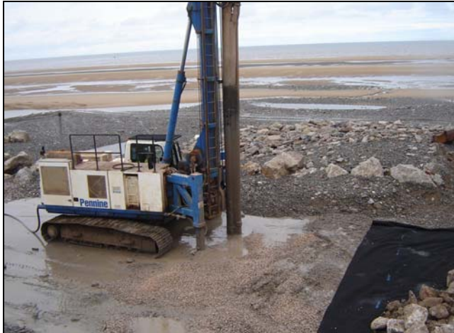
The vibro stone column piling rig in place on the beach.
