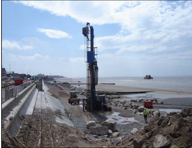
Full length view of the phase 4 site.
