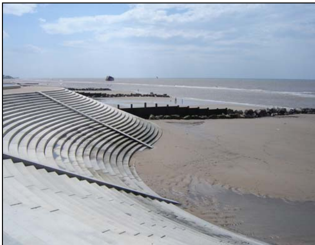
Toe of the revetment.
