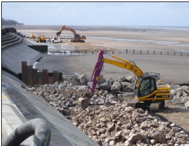
Rip rap being placed over the stone column piles.
