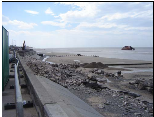
Rip rap tipping point.
