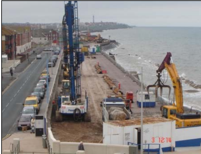
Full length view of the phase 4 site.
