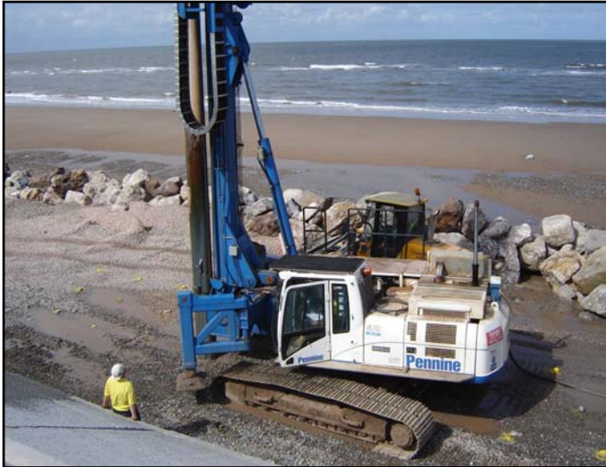
The vibro stone column piling rig in place on the beach.
