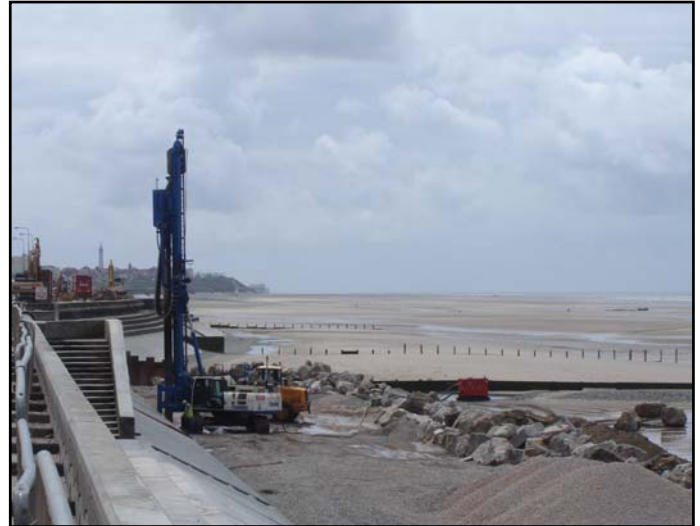
Ground stabilisation works.
