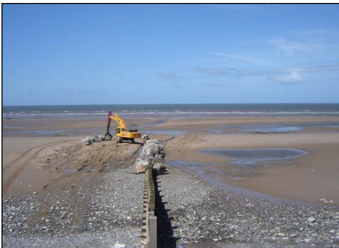
Rock armour in place along the groyne.
